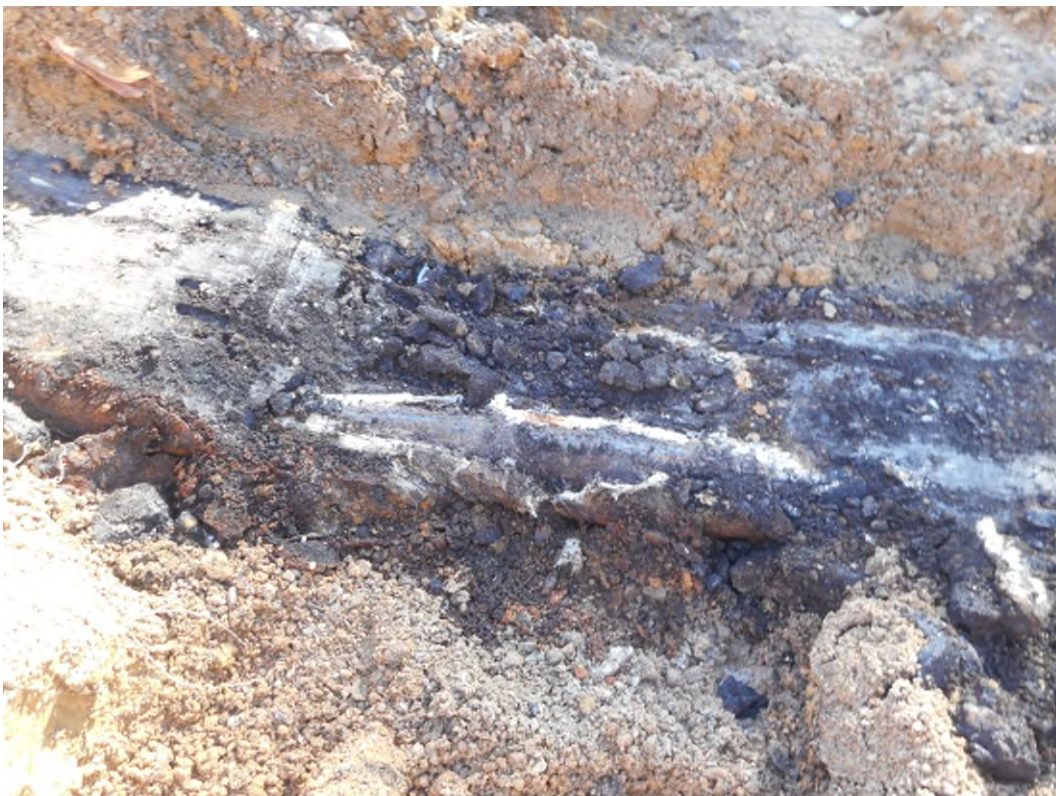
Photograph 10: Example in-ground ACM lagged heating pipes.
