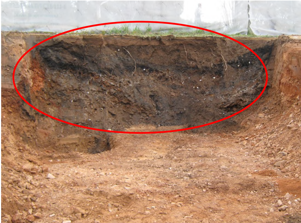
Photograph 1: Example of discoloured or stained soil.
