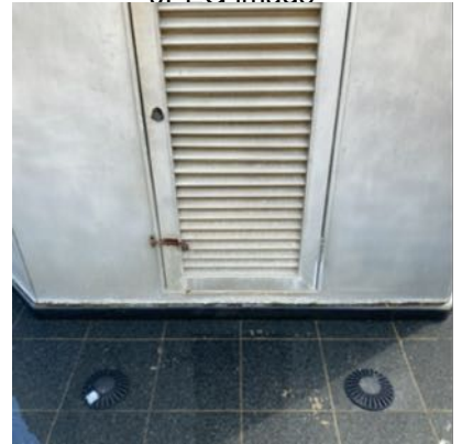
AAM Nov 2020 Podium and tower exterior 25112020~90.jpg .JPEG image
