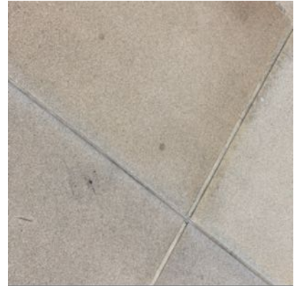
AAM Nov 2020 Podium and tower exterior 25112020~87.jpg .JPEG image
