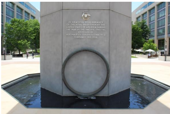
Figure 3.9 Base of the column showing the octagonal moat, large bronze wreath, dedication and sandstone paving.
