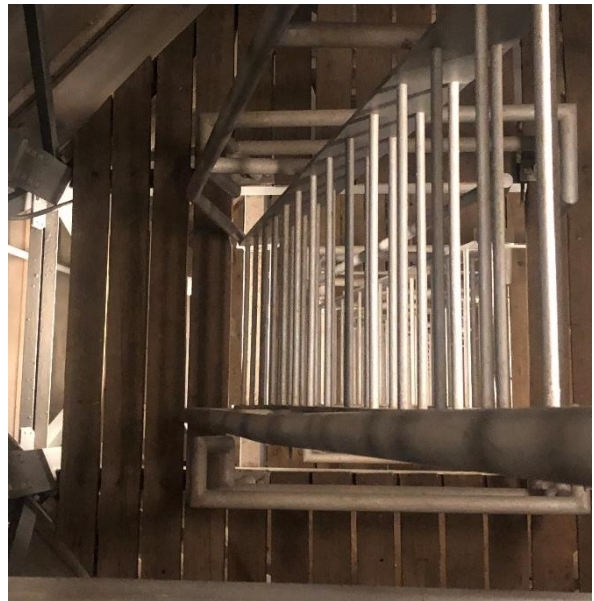
Figure 3.16 Looking down at a typical timber platform and stair system that fill the interior of the column space.
