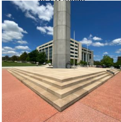
AAM Nov 2020 Podium and tower exterior 25112020~61.jpg .JPEG image
