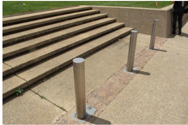
Figure 3.3 Pebblecrete steps located centrally along the southwestern boundary and stainless steel, retractable bollards.
