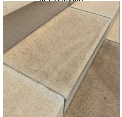
AAM Nov 2020 Podium and tower exterior 25112020~84.jpg .JPEG image
