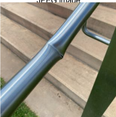
AAM Nov 2020 Podium and tower exterior 25112020~66.jpg .JPEG image
