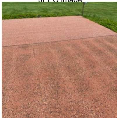
AAM Nov 2020 Podium and tower exterior 25112020~43.jpg .JPEG image
