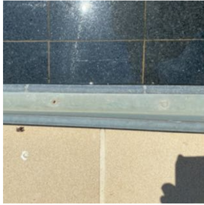
AAM Nov 2020 Podium and tower exterior 25112020~22.jpg .JPEG image
