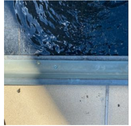
AAM Nov 2020 Podium and tower exterior 25112020~23.jpg .JPEG image
