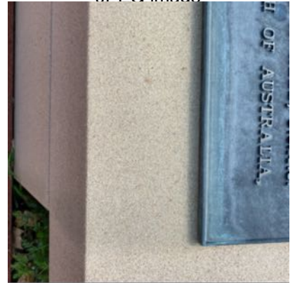
AAM Nov 2020 Podium and tower exterior 25112020~78.jpg .JPEG image
