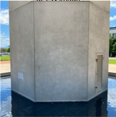
AAM Nov 2020 Podium and tower exterior 25112020~24.jpg .JPEG image
