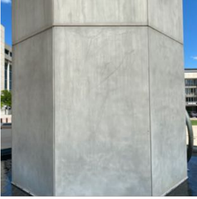
AAM Nov 2020 Podium and tower exterior 25112020~97.jpg JPEG image
