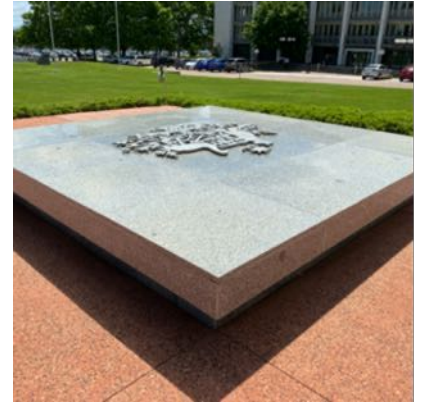
AAM Nov 2020 Podium and tower exterior 25112020~59.jpg .JPEG image
