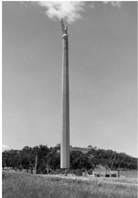
Figure 2.7 External cladding is completed, with works continuing on the podium, November 1953. (Source: ACT Heritage Library, Ref. No. 009567)
