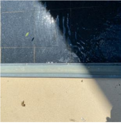
AAM Nov 2020 Podium and tower exterior 25112020~21.jpg .JPEG image
