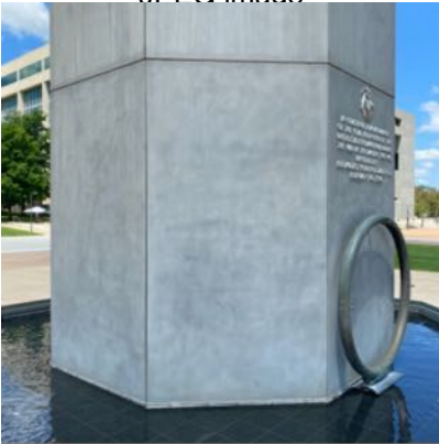
AAM Nov 2020 Podium and tower exterior 25112020~00.jpg .JPEFG image
