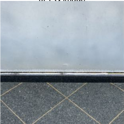
AAM Nov 2020 Podium and tower exterior 25112020~94.jpg .JPEG image
