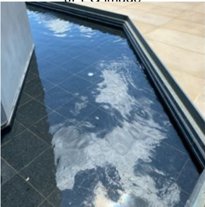
AAM Nov 2020 Podium and tower exterior 25112020~91.jpg .JPEG image
