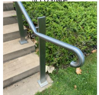
AAM Nov 2020 Podium and tower exterior 25112020~65.jpg .JPEG image
