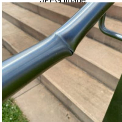
AAM Nov 2020 Podium and tower exterior 25112020~67.jpg .JPEG image
