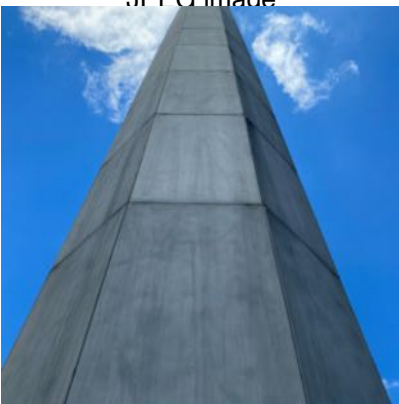
AAM Nov 2020 Podium and tower exterior 25112020~03.jpg .JPEFG image
