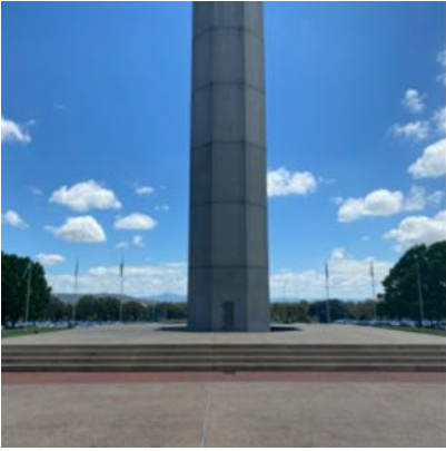
AAM Nov 2020 Podium and tower exterior 25112020~73.jpg .JPEG image
