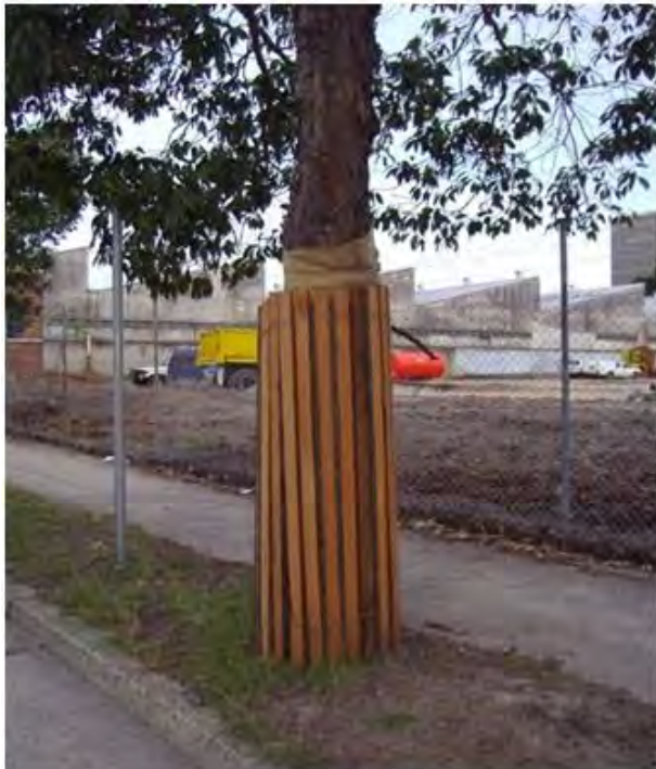
Figure 7. Example of trunk protection
