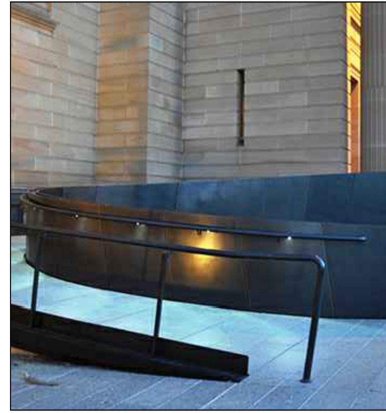
EQUAL ACCESS RAMP: WEATHERING STEEL
