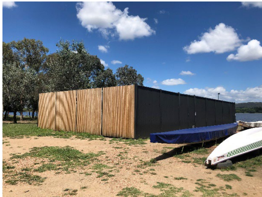
Figure 2: Temporary DBACT facility on Block 27
