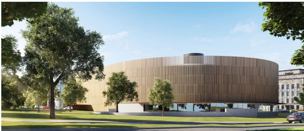
Figure 3.27 Architectural render of one of the early proposed design alternatives, showing a timber façade option. (Source: BVN Design Report, December 2021, p177)
