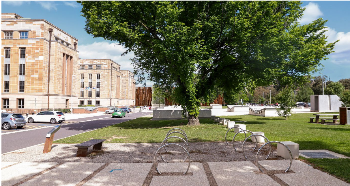
Figure 3.12 Photo montage view of the proposed building from Parkes Place East. (Source: BVN October 2022)
