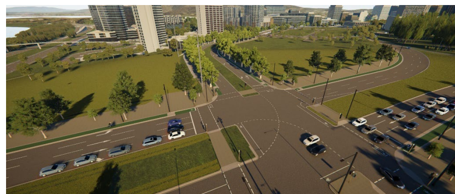
Figure 2.2 Render showing the proposed London Circuit-Commonwealth Avenue intersection, looking west towards London Circuit, City Hill is to the right. (Source: MPC, September 2021)
