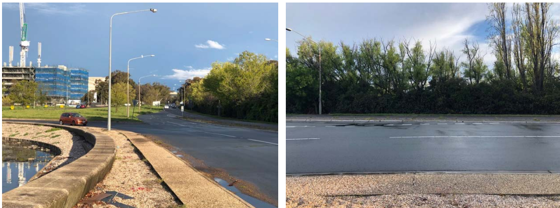
Plates 5 and 6. Views east and south from Project Site, looking to proposed extension of right turn pocket and Parliament House respectively
