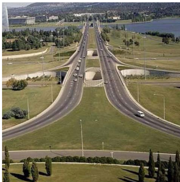
Figure 15 View south from City Hill, taken in 1975 (GML, 2021)
