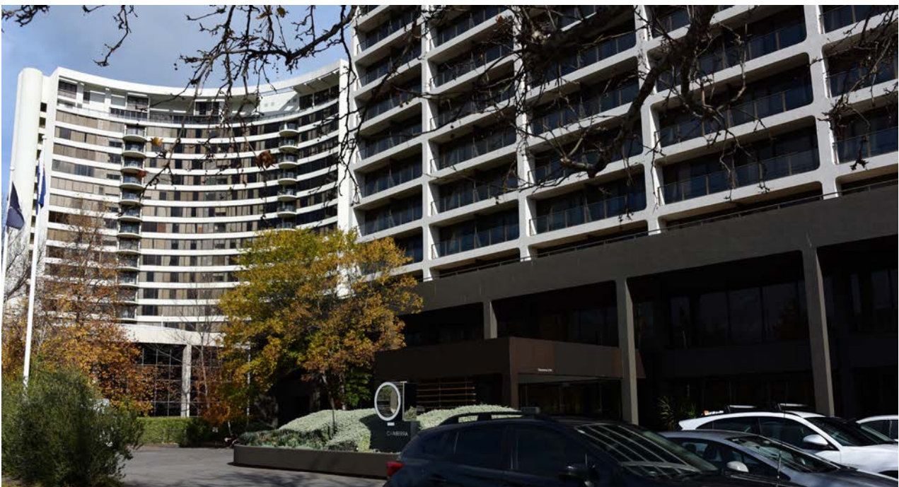
Figure 48 Taller buildings fringing London Circuit screen views to the Project from the west
