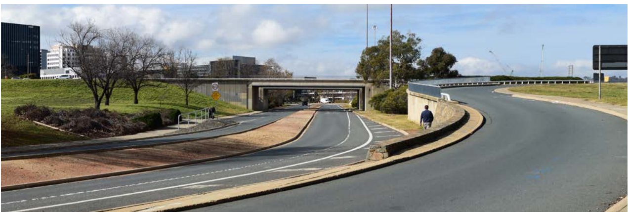
Figure 67 Detail of Figure 66 showing the view south east along London Circuit
