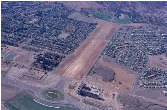
Figure 37. Aerial view of Anzac Parade looking North, under construction, c1965
