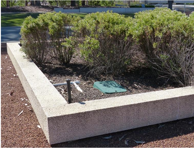
Figure 119. Irrigation infrastructure throughout the beds
