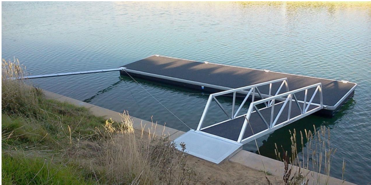
Figure 3.3 Example of pontoon to access floating sauna building. (Source: NCA)
