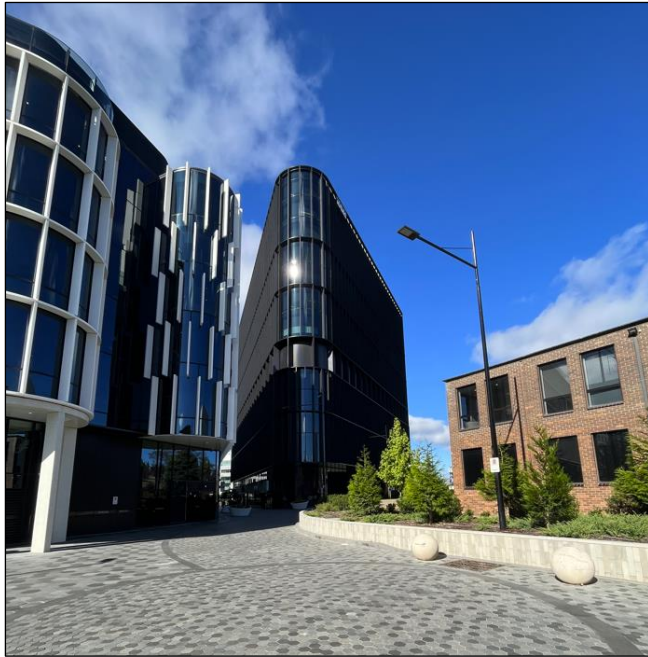
Photograph 17: 1 Constitution Avenue / 220 London Circuit as viewed from Knowles Place
