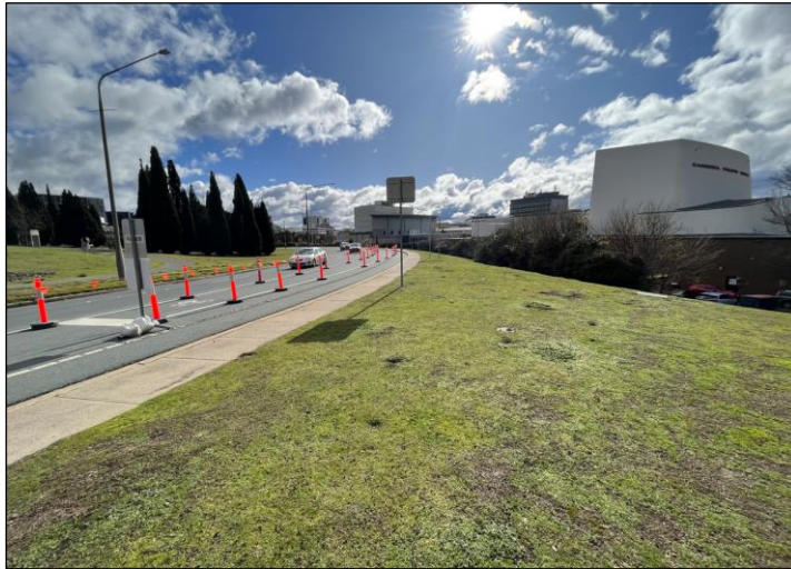
Photograph 9: Block 40 frontage to Vernon Circle looking north to Canberra Theatre.
