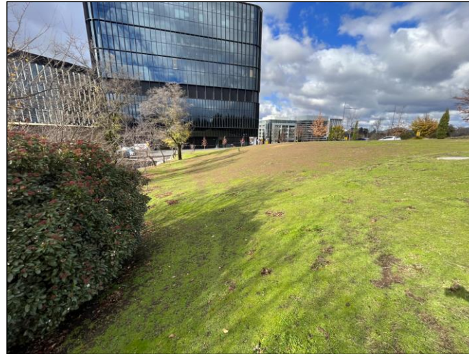
Photograph 2: Block 40 as viewed looking east towards Knowles Place and 1 Constitution Avenue.
