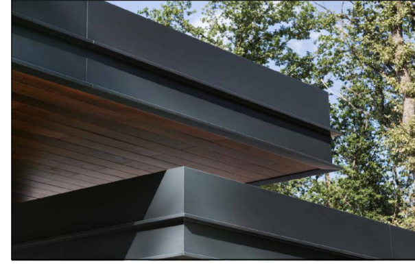
FASCIA & FLASHING - ZINC HORIZONTAL PROFILE
