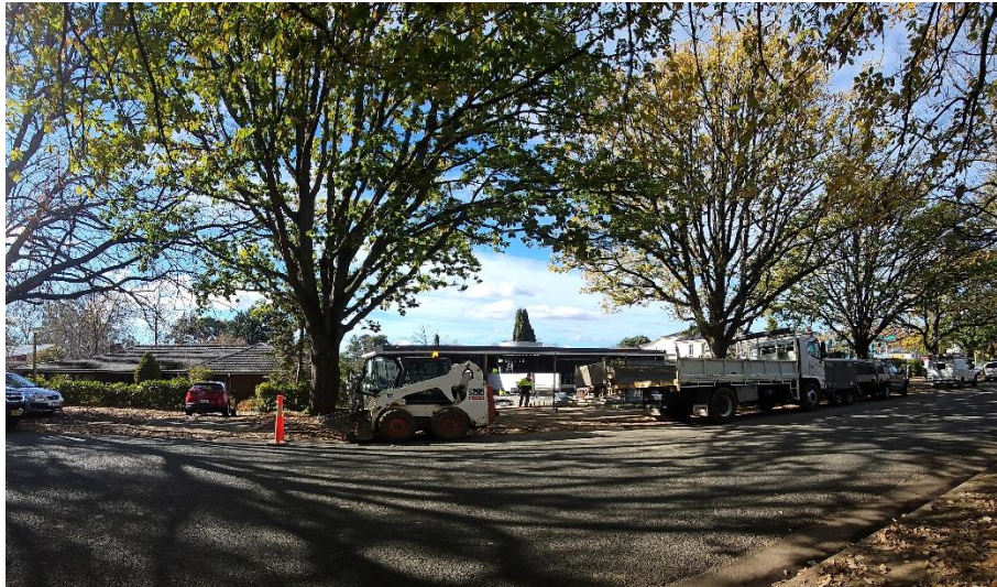
Pic 1 Re- developed Block 16 – 75 National Circuit, Modern façade with metal and concrete as primary façade material
