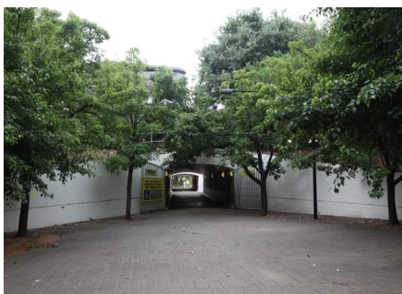
Eastern pedestrian tunnel under Parkes Way
