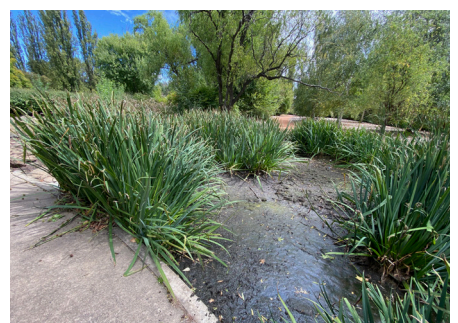
Silted up Marsh Gardens - recently addressed
