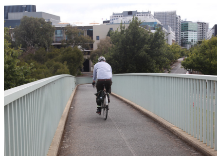
Narrow footbridge to City over Parkes Way
