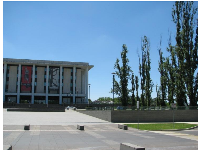
Figure 9 The walkway down the central axis of the forecourt showing the slope and the retaining wall that creates a near level planting area for the poplars.
