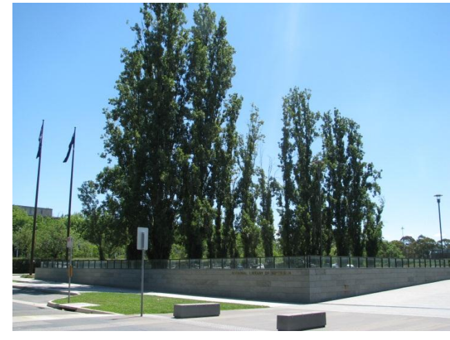
Figure 10 The NE corner where the retaining wall is highest, the trees suffered more root loss during the wall replacement and the trees are suffering most.
