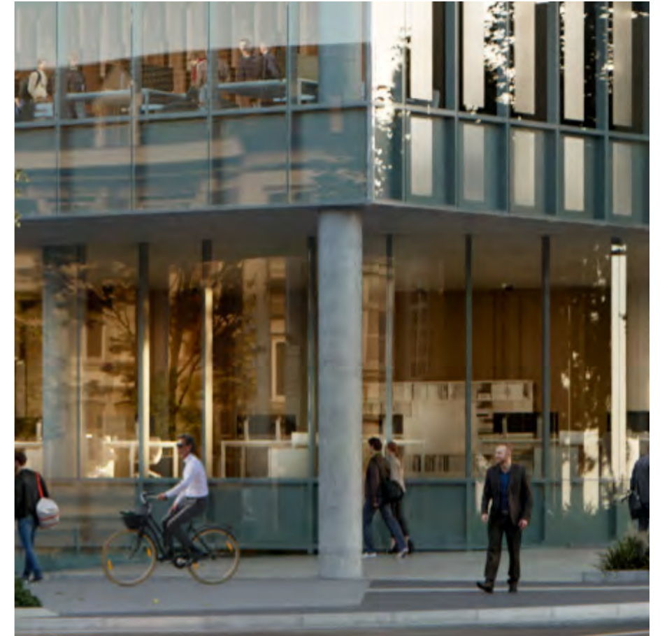
NATURAL CONCRETE FINISH TO COLONNADE COLUMNS
