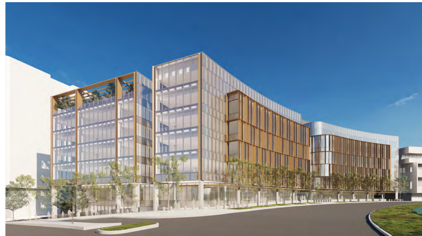
Revised building massing with facade addressing site and street alignment. Image also shows updated response to solar control to the east elevation with revised density to the screening element with the addition of frits to areas without physical sun and privacy protection measures.
