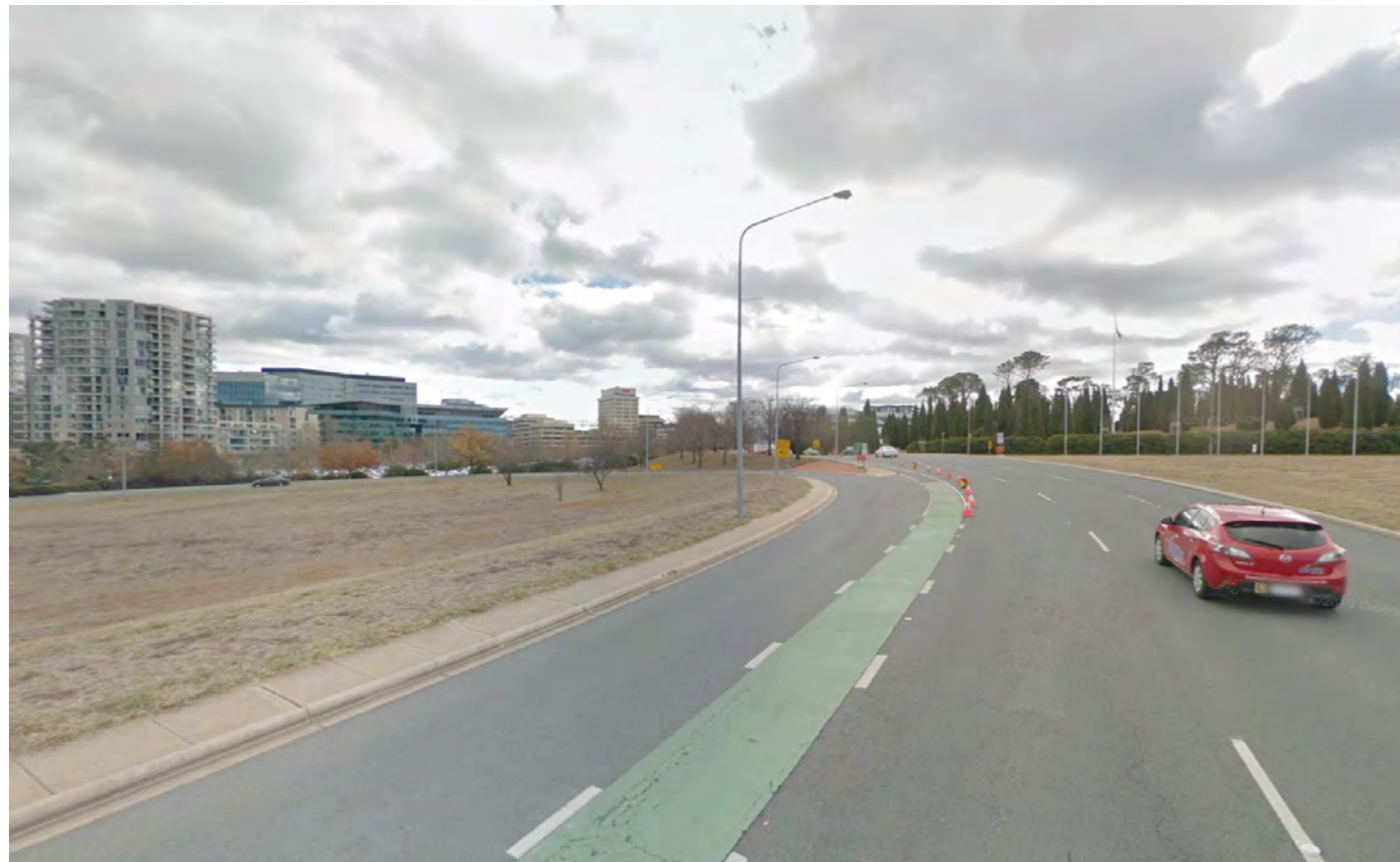
SOUTHERN APPROACH FROM DISTANCE
