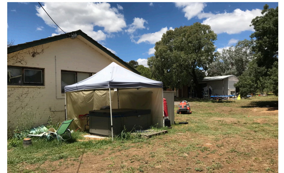
View 6 - Rear of cottage and side of Curtin Budget Motel
