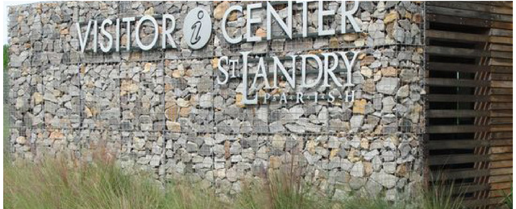
Feature Walls with Signage
