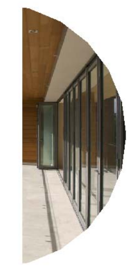
AGWS1 - ALUMINIUM GLAZED WINDOW SUITE - TYPE 1 ALUMINIUM FRAMED WINDOW SUITE - POWDER COATED - WINDSPRAY (GREY). CLEAR GLASS.
