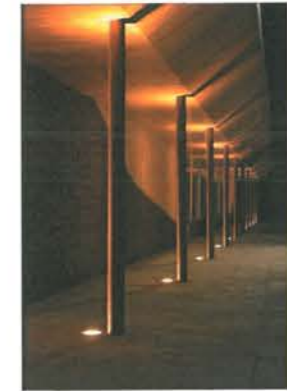
IN GROUND UPLIGHTERS TO COLUMN BASES
