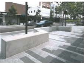
PRECAST CONCRETE BBQ BENCH - OXIDE FINISH / STEEL ACCESS PANELS / STAINLESS STEEL HOTPLATE AND SINK
