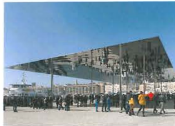
MIRROR FINISH SOFFIT
