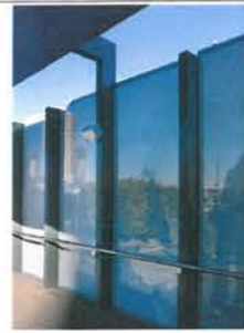
STEEL FRAMED PORTAL
