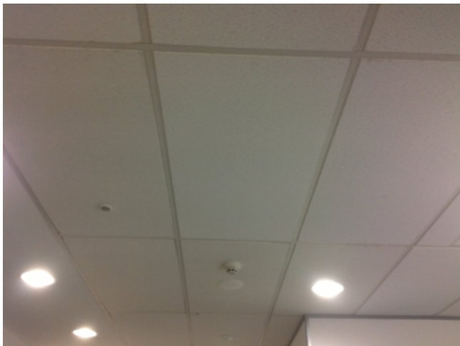
Photo No: J123625-003-CEN-779 Result: SMF - Positive Building/Level: Office Block-Level 1 Room/Location: Office Areas-Throughout Feature/Material: Ceiling Tiles-Compressed Ceiling Tiles
