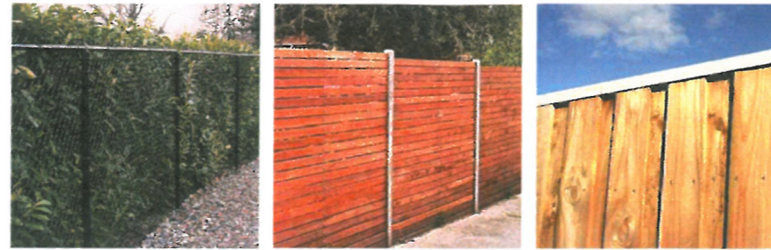
FT1: 1000mm Transparent Fencing FT2 - 1800mm Timber Fencing FT3 - 1800mm Site Boundary Fencing
