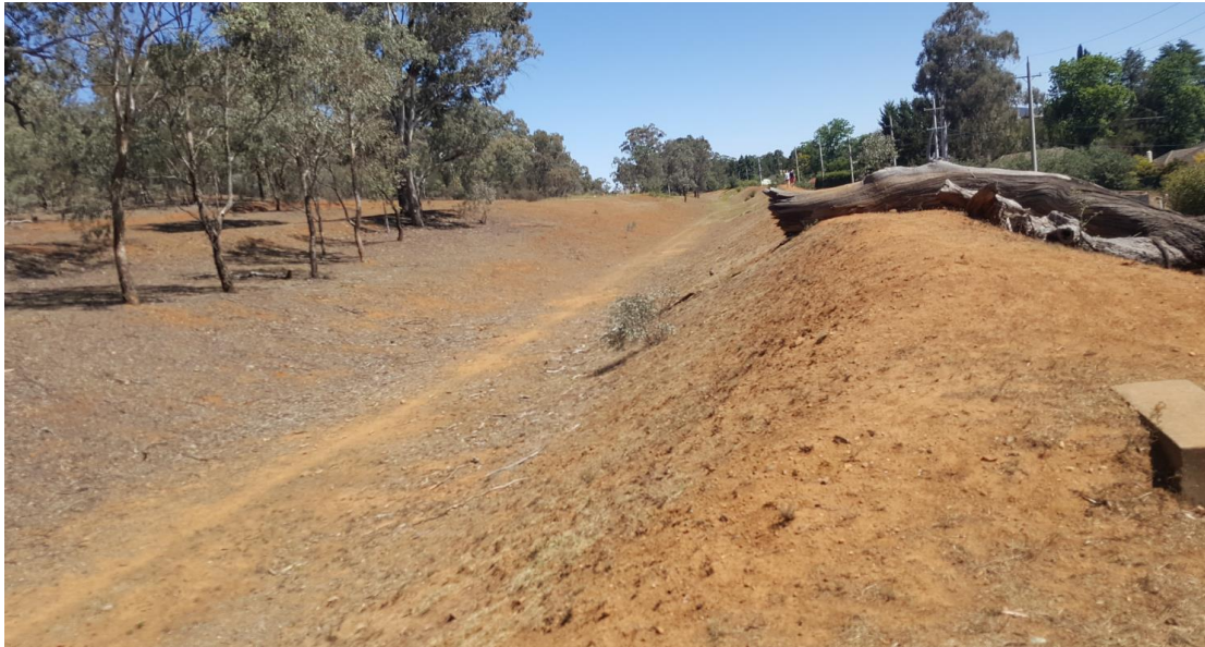
Figure 5 – Red Hill cut-off swale
