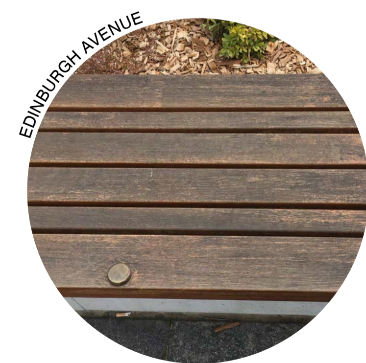
Timber batten tops
