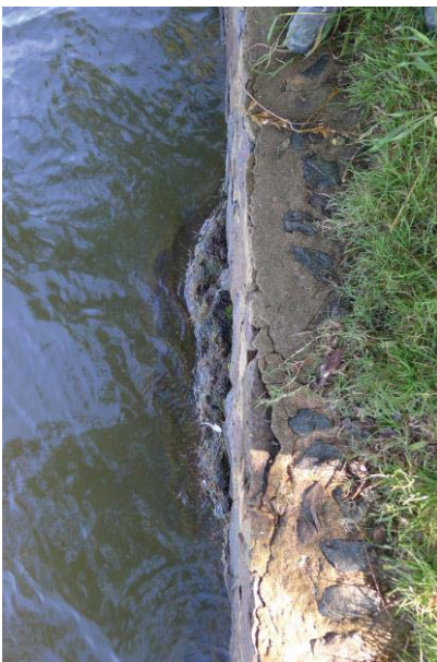
Figure 6 - Examples of root growth through the lake wall
