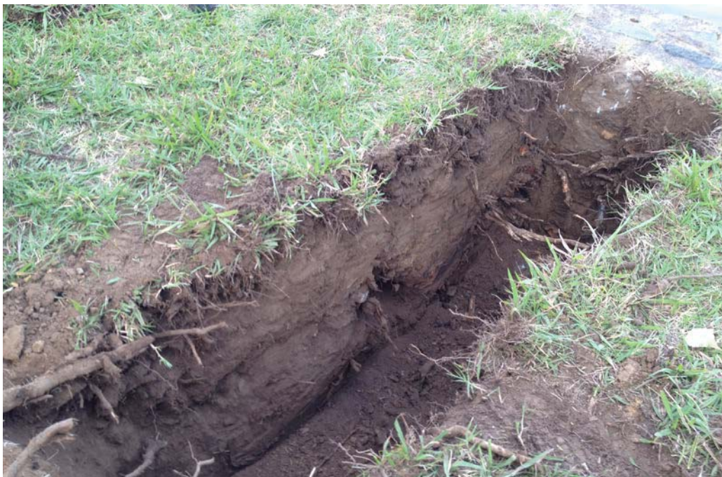
Photo 8 – View of southern pit wall of Pit 2
